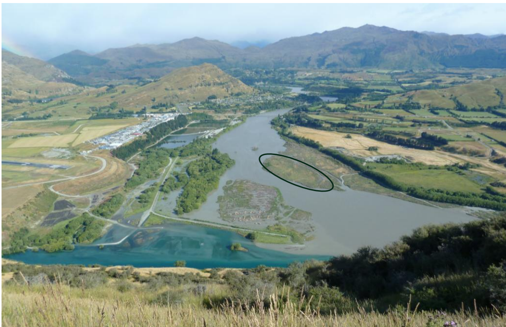
Figure 12: A flooded Delta at around 400m 3 /s following a peak of over 500m 3 /s after the construction of the RESA and Flood Retention Wall and the clearance of willows from the Delta islands. The gravel removed to build up the ground level of the Shotover Country subdivision is indicated.
